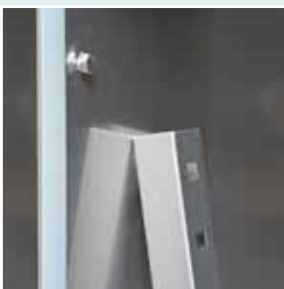
Removable shelf supports for deep cleaning
